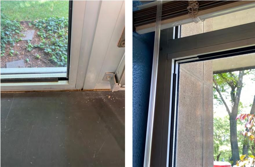
The aluminum and single pane glazing is original to the building and requires replacement as the glazing compound (asbestos containing) and perimeter caulking (asbestos containing) are failing and for improved thermal / energy efficiency. All of these windows are under contract to be replaced this fall (2021) and therefore the costs are excluded from this report.
